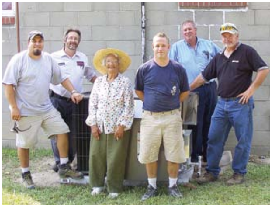
Alice Watkins poses with the NAOHSM volunteers who installed her new Thermo Pride3 ThermoPack. They are, left to right, Dave Porter, Phillips Energy; Filmore Brinkley, E.T. Lawson; Bill Alcombrack and Lee Mershon, Phillips Energy; and Gene Vickhouse, Cutting Edge Total Comfort.
