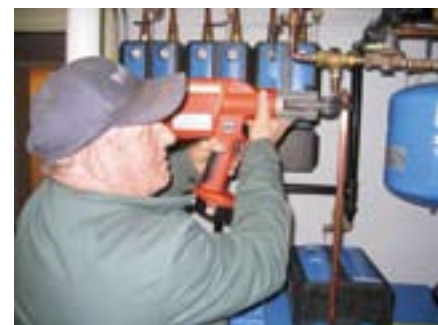
Bill Lacey demonstrates the Viega ProPress pipe-joining system.
